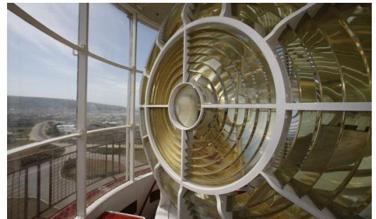
Cape Agulhas Lighthouse's 1 st order traditional lens, producing a light of 7.5 million candela that can be seen at a distance of 31 nautical miles (57 km)
