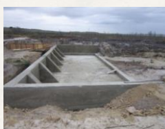
Ratel River structure
